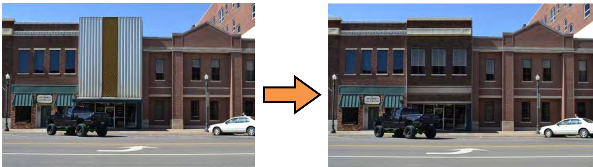
Figure 4.4 521 Commercial Street. Façade material replacement and window restoration.
